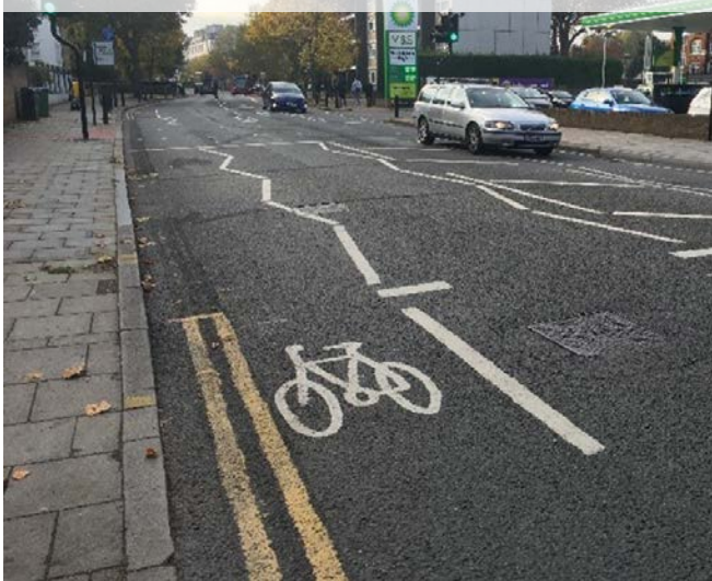
Figure 6.19: Zig-zag markings placed away from the kerb to continue cycle lane, Greenwich
