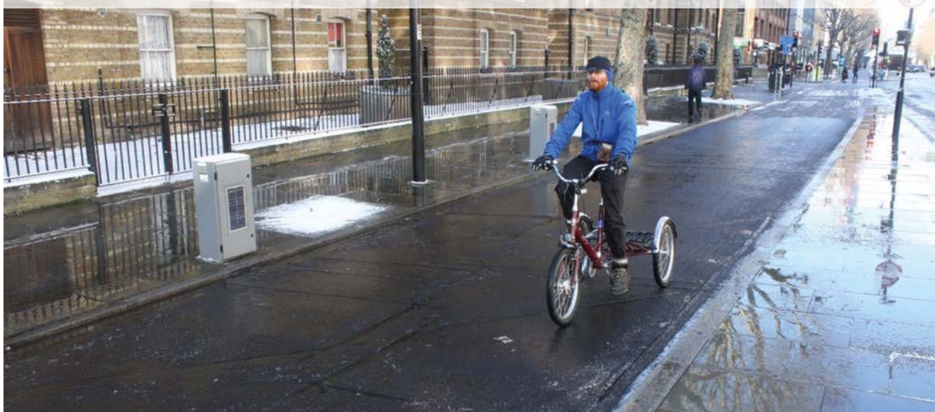
Figure 6.5: Intermediate level cycle track, with level difference to footway and carriageway, London
