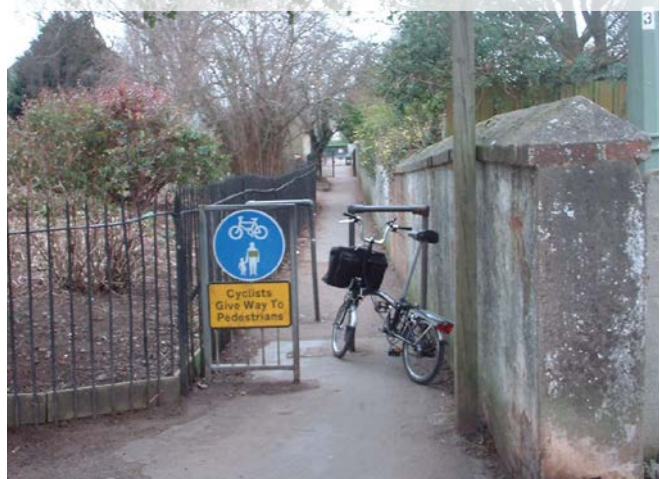
Figure 1.8: Barriers to cycling along a shared-use route (note yellow sign is not permitted in TSRGD)
